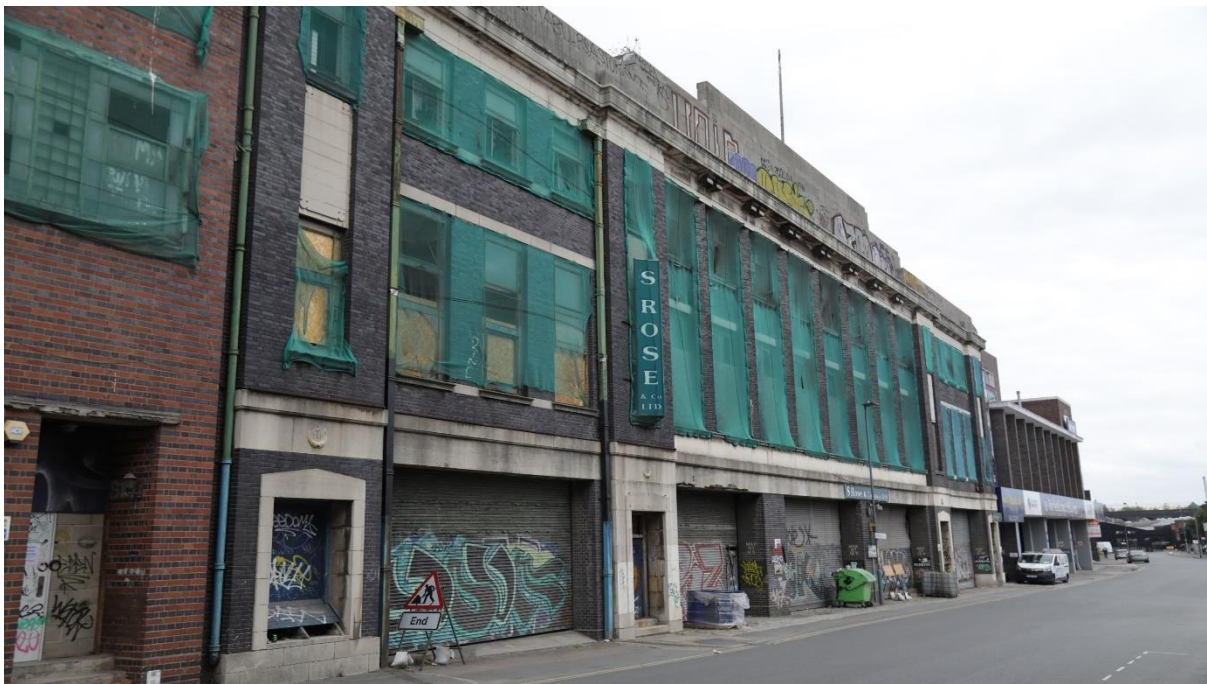
Image: 'Before' image of the Typhoo factory in Digbeth, Birmingham that is being redeveloped for new BBC Studios, courtesy of BDP
